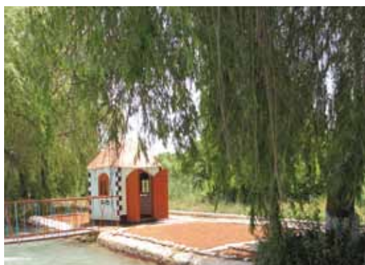
Rehabilitated hydro-post of Kyzyl-Kyr WUA.
