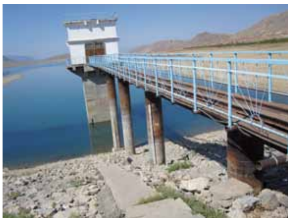
The tower outlet at Tortgul eastern dam.
