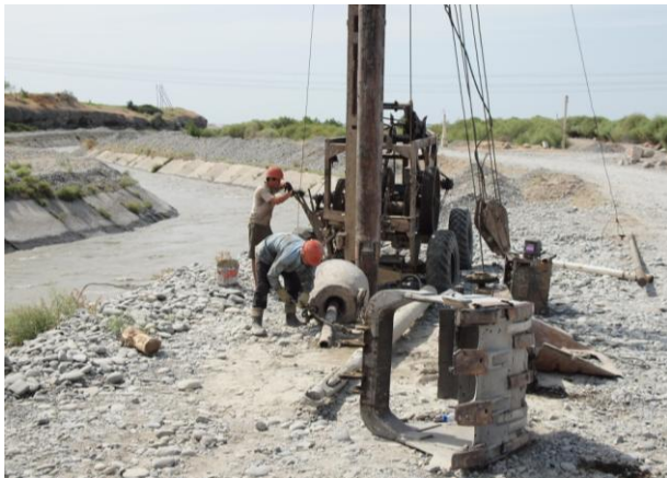
Groundwater observation bore at Ravatkhodja headwork
