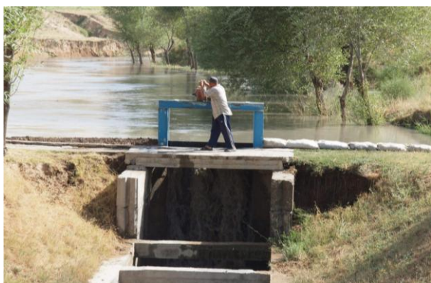
Headwork of Bad Bad irrigation canal
