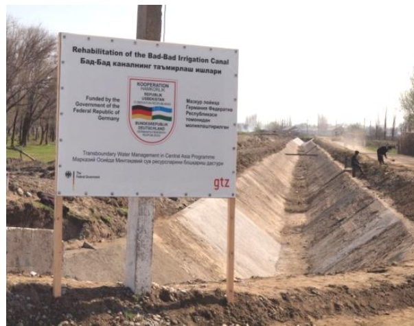
Rehabilitation works at the canal
