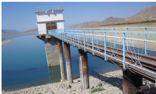
The tower outlet at Tortgul eastern dam
