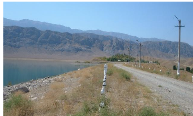
The crest of Tortgul western dam
