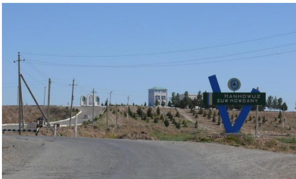
Entrance to Khanhovuz Irrigation System
