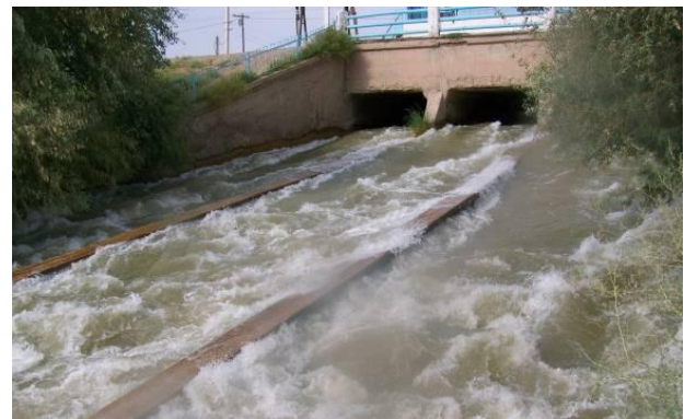
Khanhovuz irrigation canal
