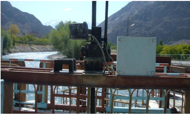
A flat gate hoist mechanism in the main body of Isfara headwork
